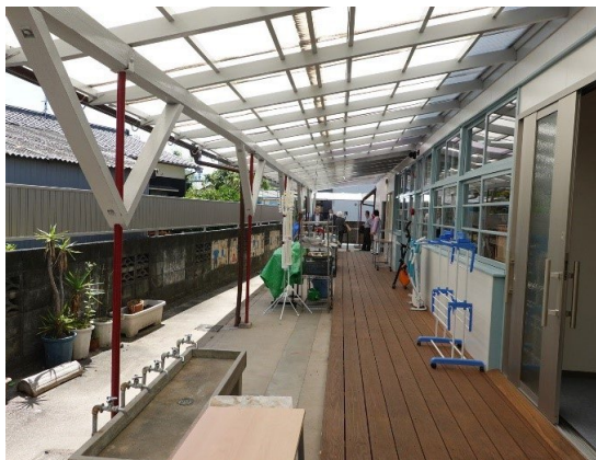
WELL 旧園舎外廊下
